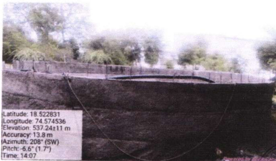
Photos of Boar Well/Open well Recharge
